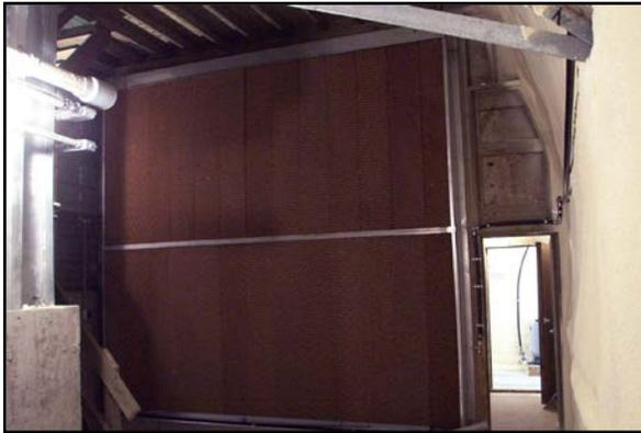
**Figure 26.** An evaporative cooling pad is constantly saturated with water while air is moved through the pad to provide humidity and cooling to potato tubers in storage.
