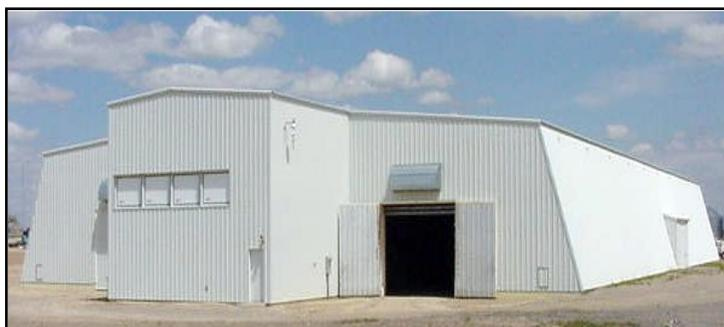
**Figure 24.** Modern potato storage facilities used to store potatoes in northern potato-production areas. Storage capacity can range from 500 ton to over 20,000 ton. Storage facilities are generally insulated and equipped with a forced-air ventilation system to control temperature and humidity. Most potatoes are stored in bulk piles, but box storages are utilized in some areas. (W. Bohl)
