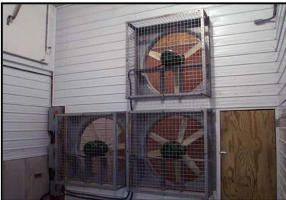
**Figure 25.** Modern potato storage facility with axial flow fans used to move air from the fan room to the lateral distribution ducts to maintain a constant temperature of the potato tubers.
